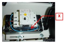
5. Unscrew and open the housing of the main switch (4) with the Phillips screwdriver (N). The blue cable link (X) can be seen running from the upper left to the lower right.
