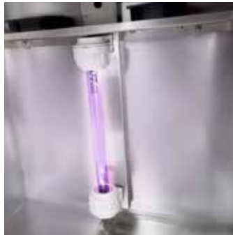
Air UV recirculation system in the chamber
